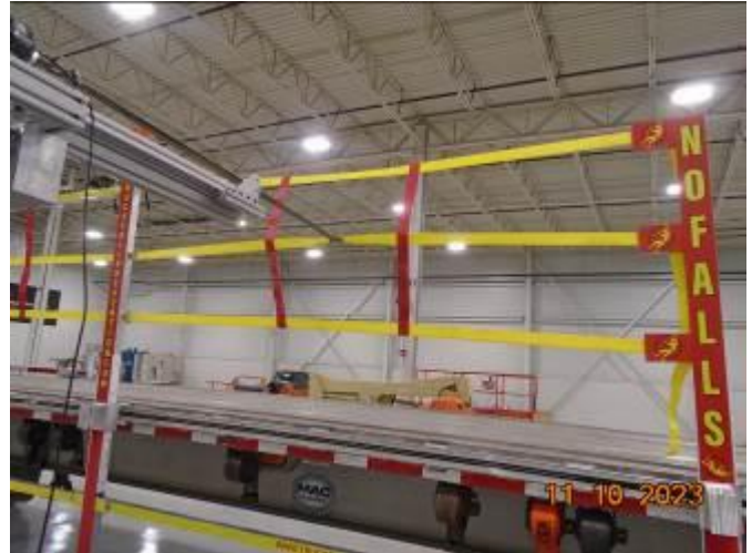
Figure 21: Right-middle under load
